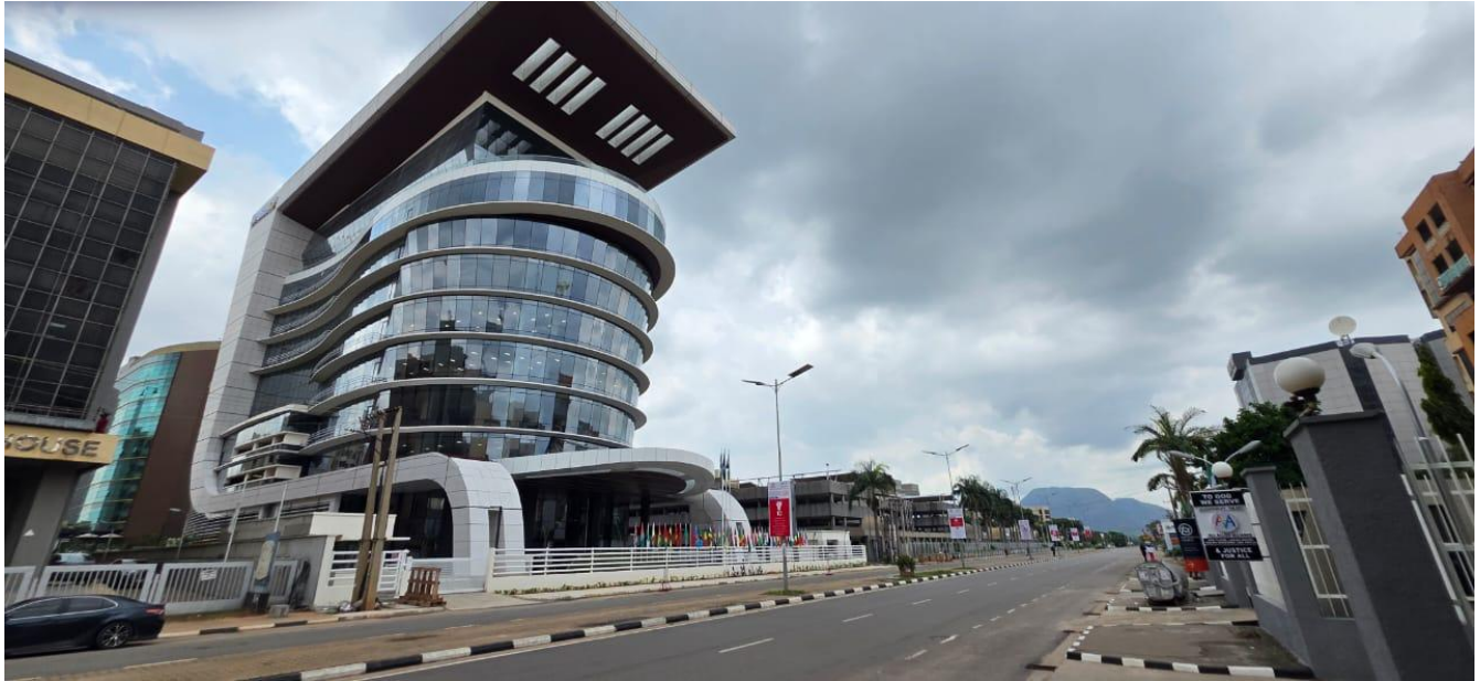
New Africa Re headquarters, Abuja
