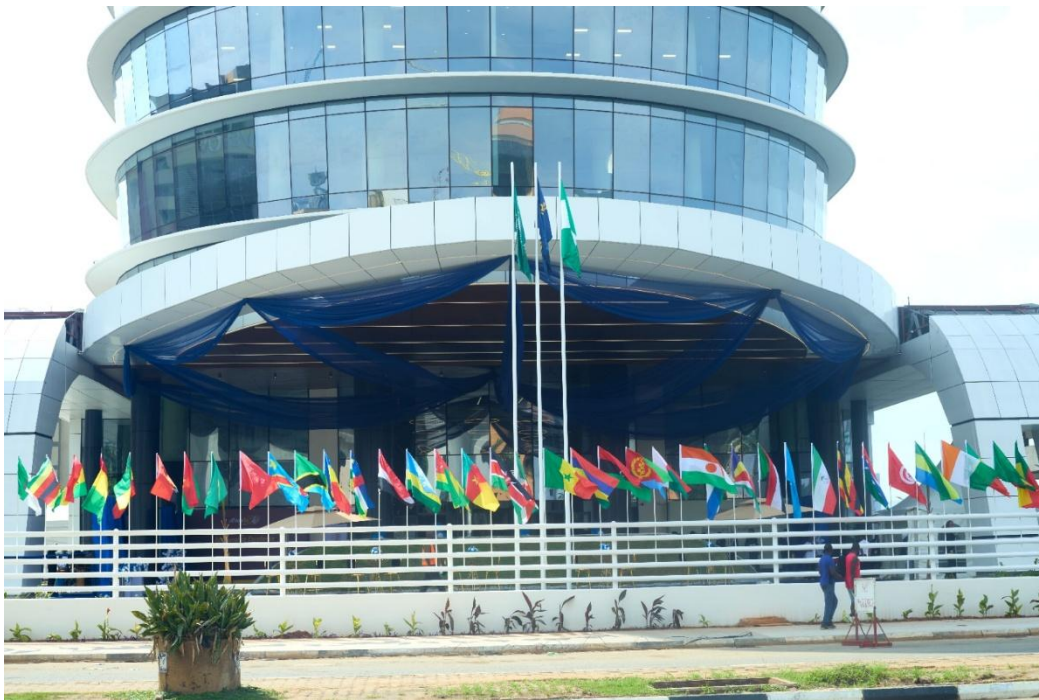
New Africa Re headquarters, Abuja
