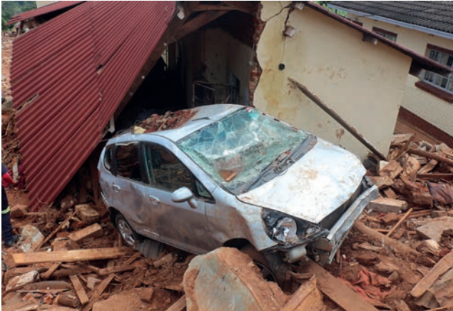
Cyclone Idai aftermath
